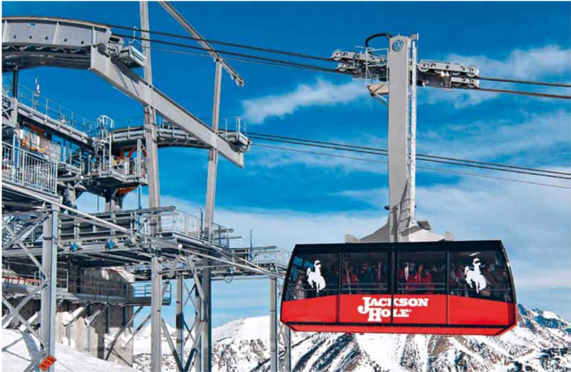
Figure 3.4.2-1 Doppelmayr/Garaventa Aerial Tramway, Jackson Hole, WY USA (Image: Doppelmayr/Garaventa)
