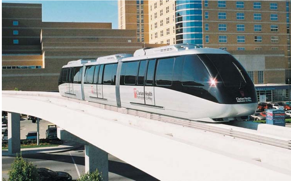
Figure 3.1.5-1 Schwager Davis UniTrak, IU Health, Indianapolis, IN USA (Image: SDI)
