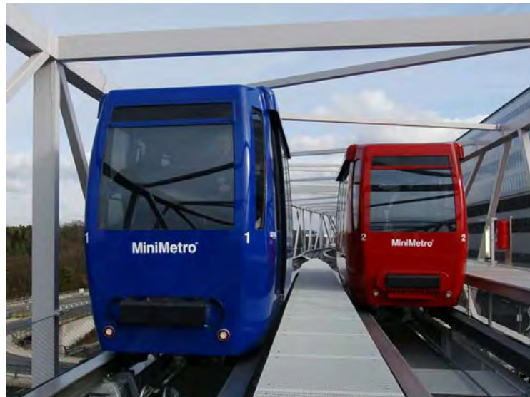
Figure 12. Leitner-Poma Mini Metro small vehicle on The Squire metro, Frankfurt Airport, Germany 11
