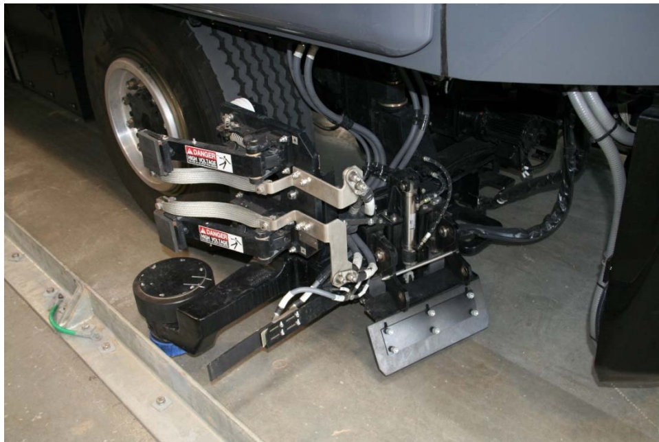
Figure 3.1.4-6 Mitsubishi Crystal Mover guidance system, Atlanta Airport, GA USA (Image: Lea+Elliott)
