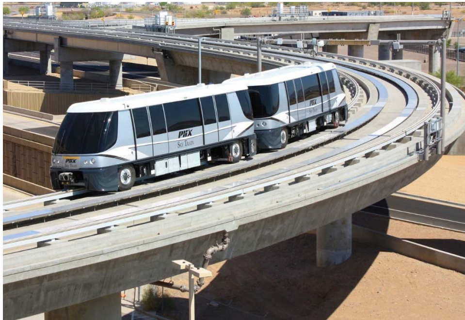
Figure 3.1.2-2 Bombardier INNOVIA APM 200, Phoenix Airport, AZ, USA (Image: City of Phoenix)
