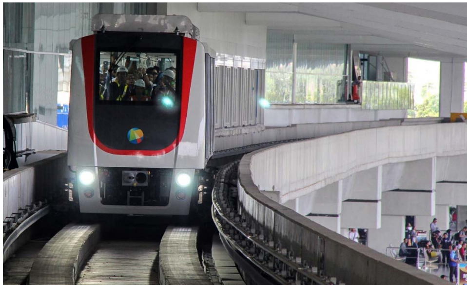
Figure 3.1.7-2 Woojin Advanced K-AGT, Jakarta Airport, Indonesia (Image: Jakarta Post)
