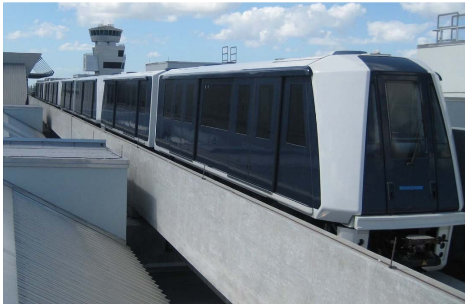
Figure 3.1.4-2 Mitsubishi Crystal Mover, Miami Airport, FL USA (Image: Lea+Elliott)
