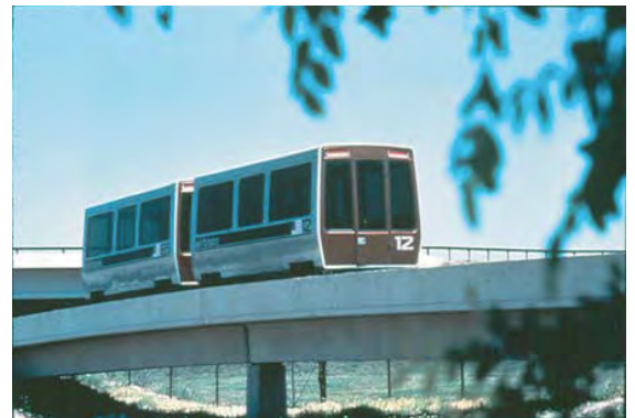
Figure 3. Dallas/Fort Worth International Airport AIRTRANS 3
