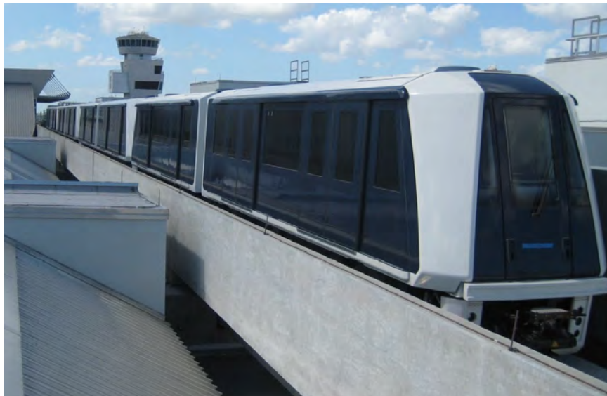
Figure 5. Mitsubishi Crystal Mover, Miami Airport, FL USA 5
