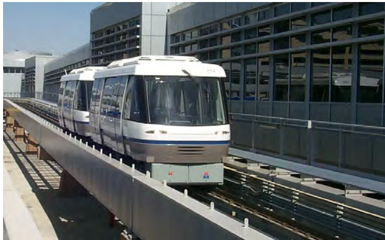
Figure 11. Leitner-Poma (formerly Poma Otis) Mini Metro utilizing steel wheels/steel rail guidance, Minneapolis-St. Paul Airport, MN USA 10
