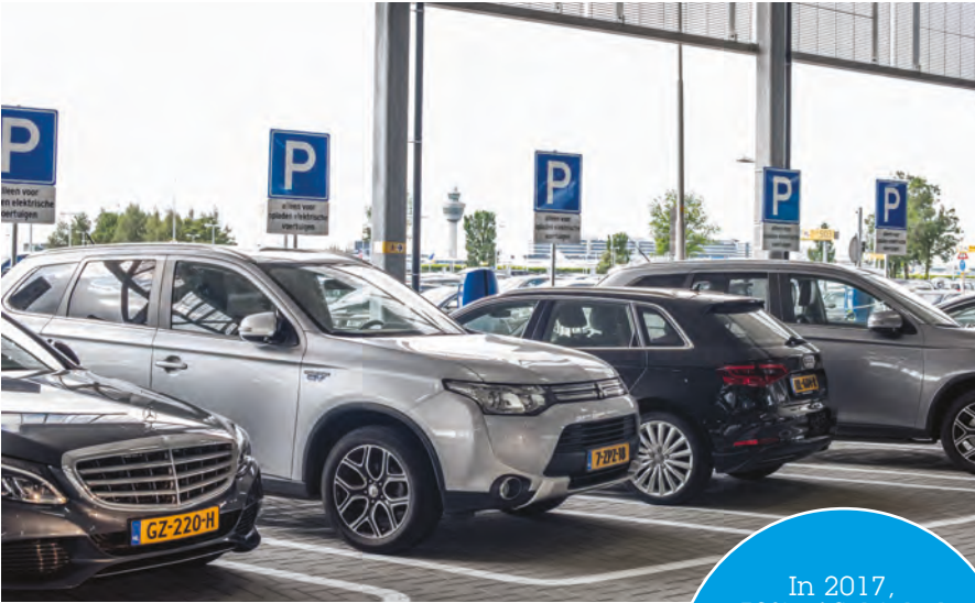
ABOVE: Electric vehicle charging points at Amsterdam Airport Schiphol
